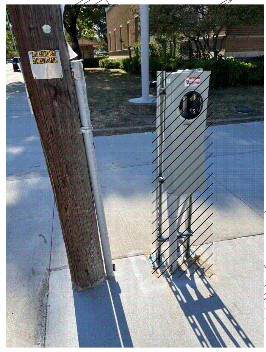
EXISTING METER PEDESTAL
