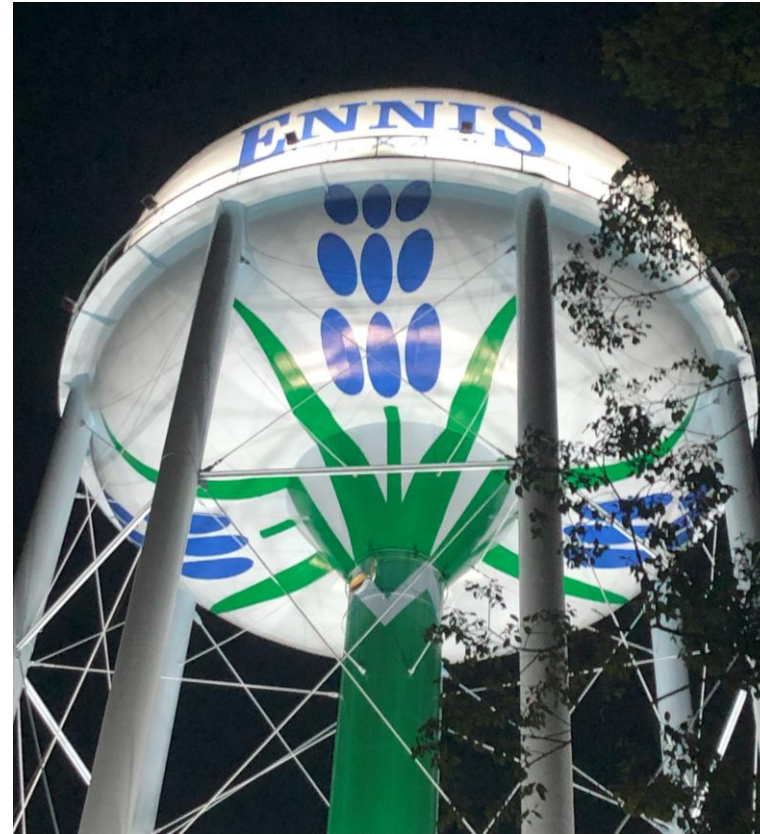
#2 Elevated Storage Tank 750,000 Gallons
