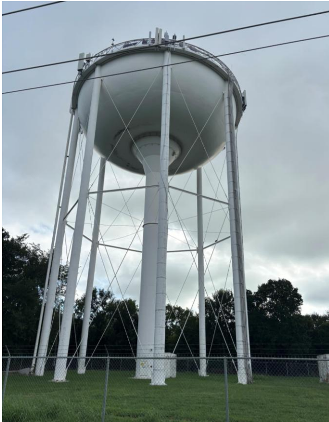
#1 Elevated Storage Tank 750,000 Gallons
